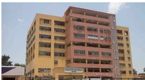
Front View Kawempe Hospital
